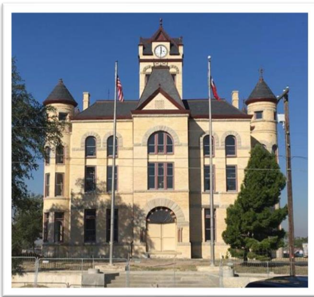
Figure 3-2: Karnes County Courthouse (after restoration)
