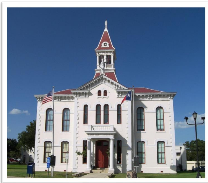
Figure 3-4: Wilson County Courthouse
